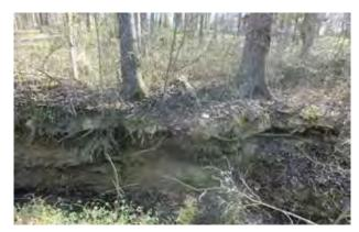
Figure 21: Improve major erosion along stream bank
