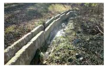
Figure 20: Remove retaining wall and restore bank
