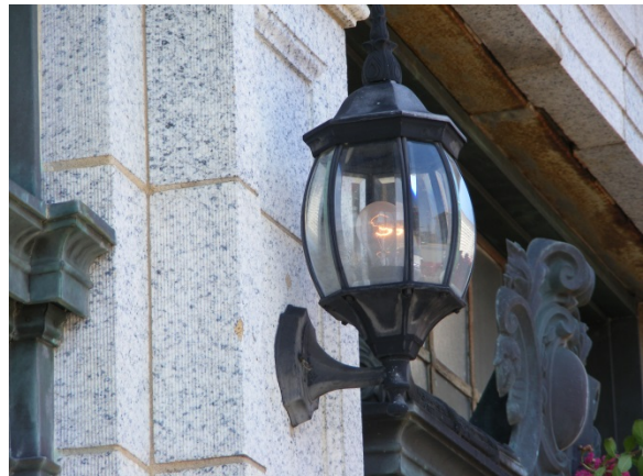
Historic light fixture. 36 SW Court Sq
