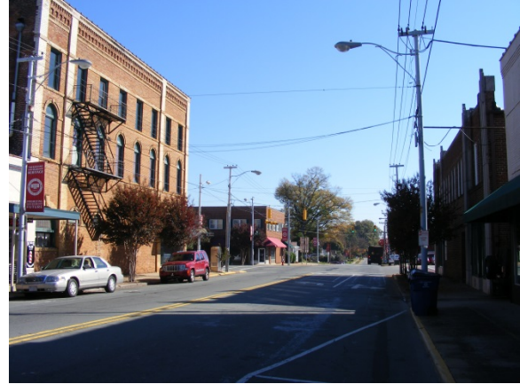
W Harden St, looking east toward N Main St
