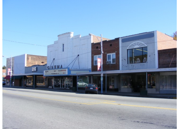
East side of the 100 block of N Main St
