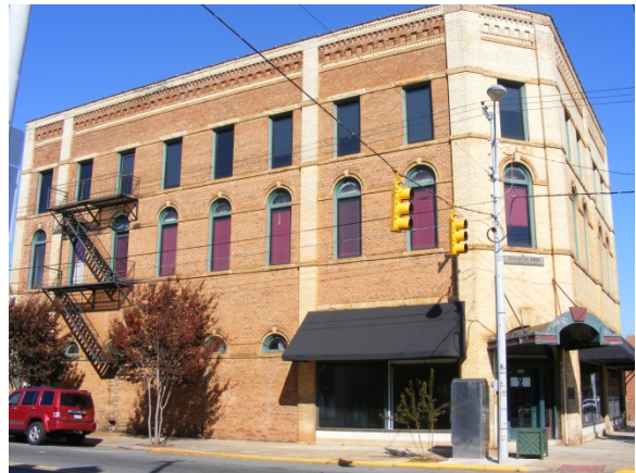
Exterior fire escapes. 200 N Main St
