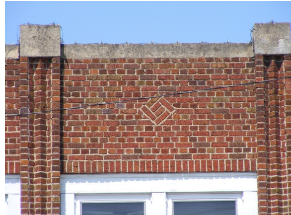
Decorative masonry detail. 142 N Main St
