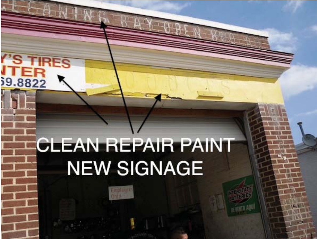
Photo 5. Facing above garage doors.
