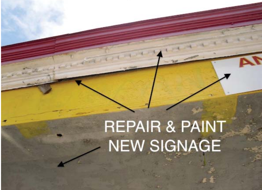
Photo 6. Canopy facing and crown modling.
