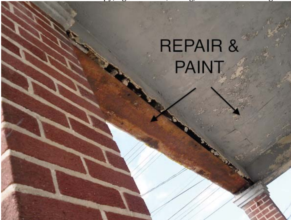
Photo 4. Underside of canopy, exposed beam, failing plaster.
