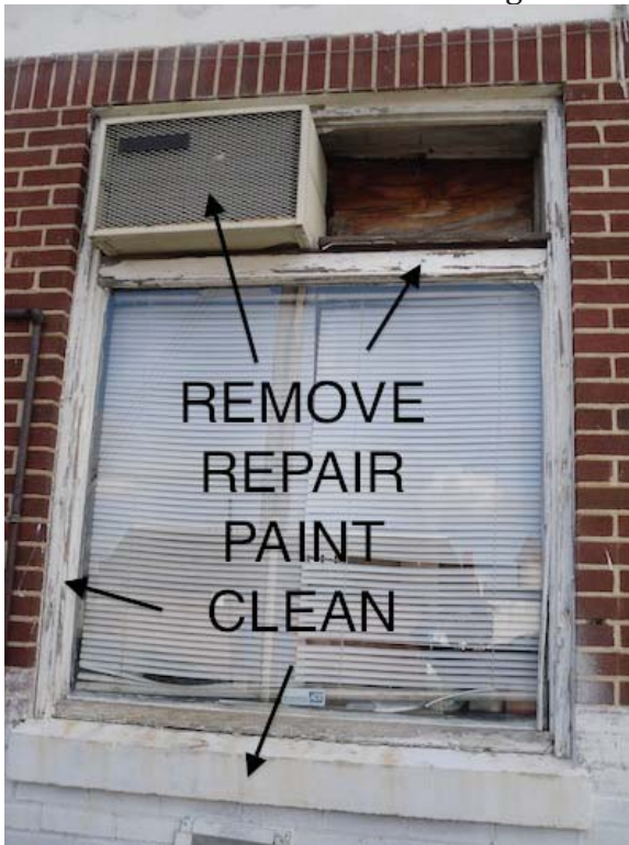
Photo 8. West side window facing, missing glass.
