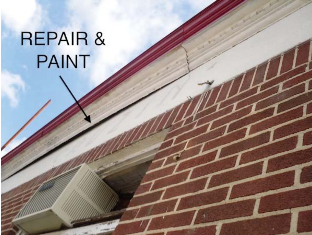
Photo 7. West side crown molding.
