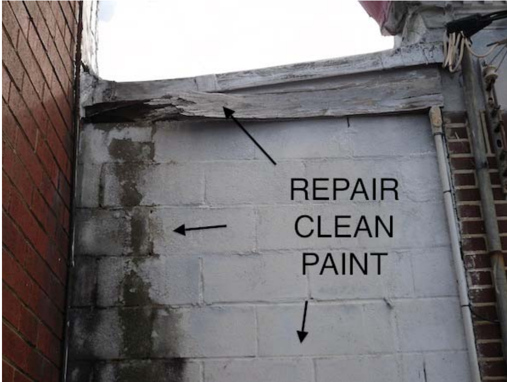
Photo 9. Rotted wood, mold on brick, water damage from roof run-off.
