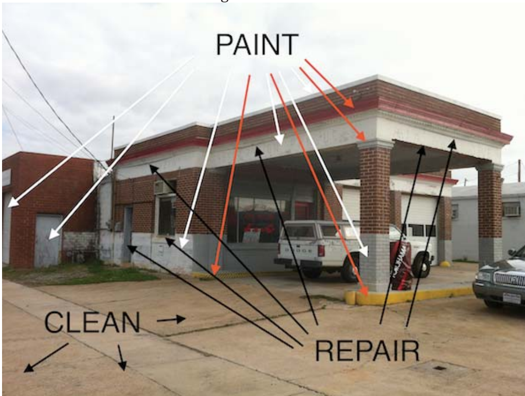
Photo 2. SW front of the building.
