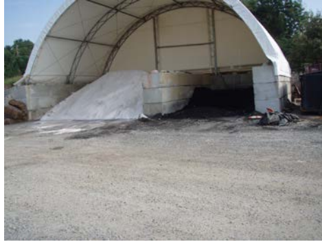
Salt Storage at Public Works
