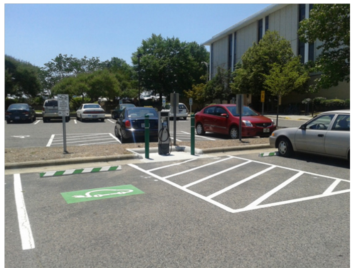
Figure 1. Accessible public charging station at the Durham County Main Library, Durham, NC.
