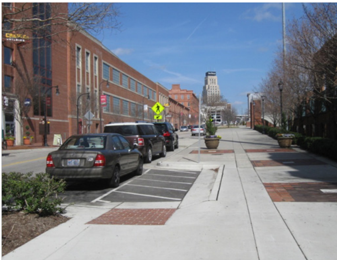
Figure 4. On-street van-accessible parking requires lots of adjacent space.
