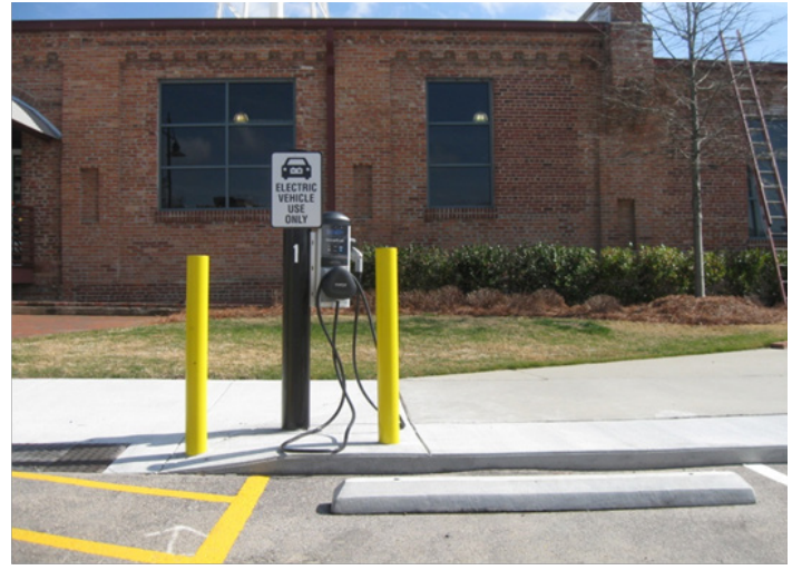
Figure 3. Over-protection can hinder accessibility of charging stations.
