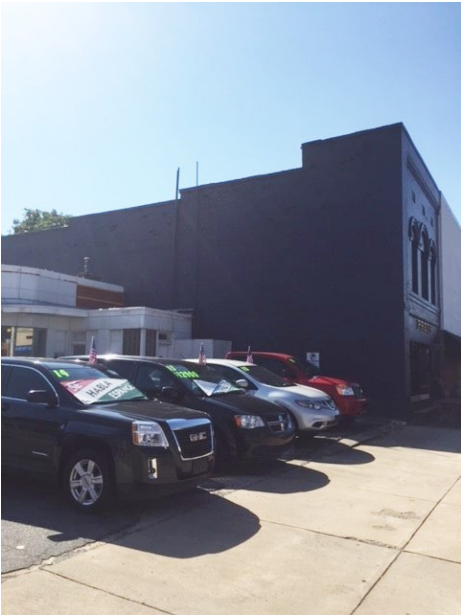
Current Facade – North Wall
