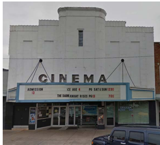
Renovations underway with the 2014-2015 and 2015-2016 Historic District Façade Grant Program. After the renovation (pictured above) and before the renovation (pictured below- image from Google Maps).
