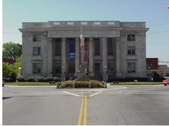
Alamance County Courthouse
