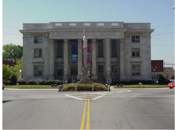
Alamance County Courthouse
