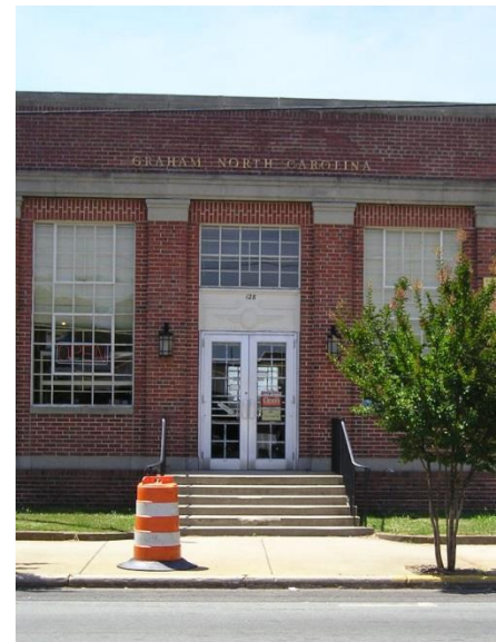
Former Post Office
