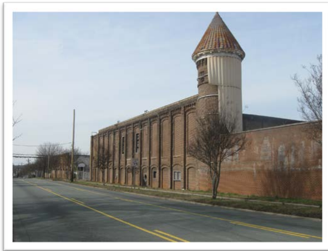
The Oneida Mills property is in the process of being redeveloped into multifamily housing. This project may serve as a catalyst for further revitalization and reinvestment in the area
