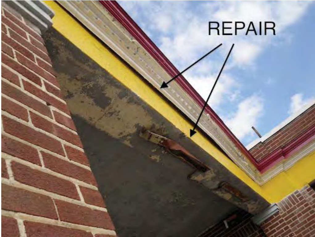
Photo 3. East front of canopy, light fixtures, facing, and crown molding.
