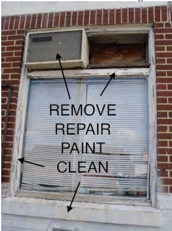
Photo 8. West side window facing, missing glass.
