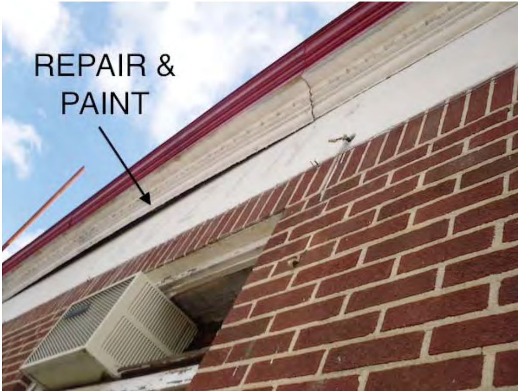
Photo 7. West side crown molding.
