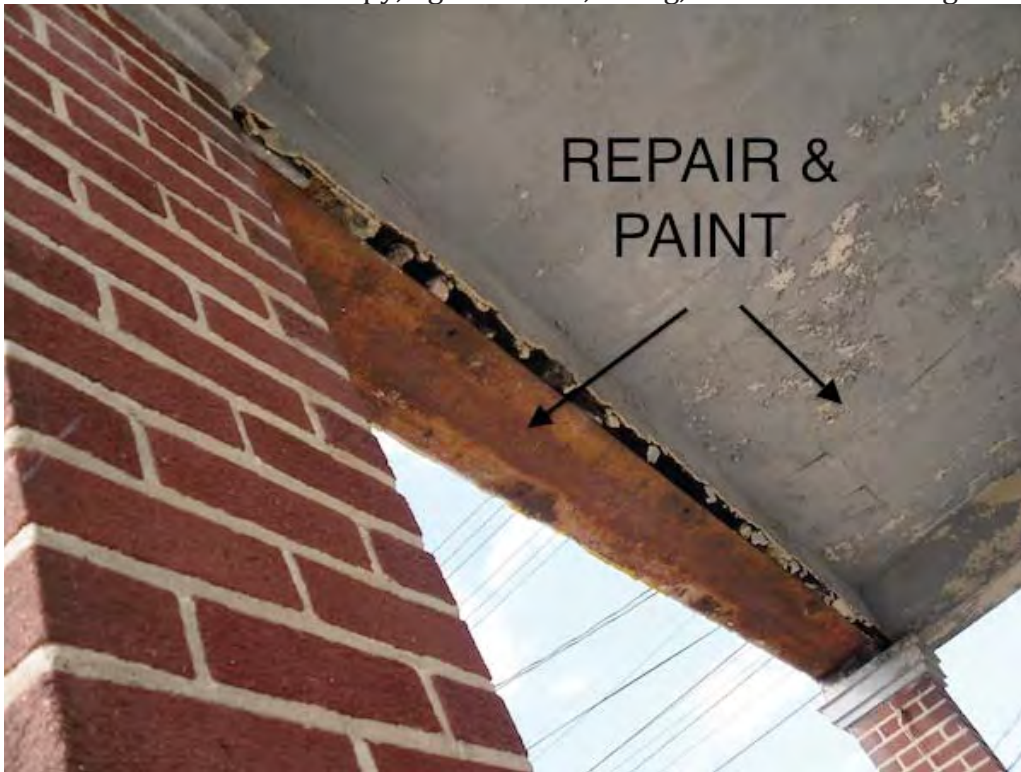
Photo 4. Underside of canopy, exposed beam, failing plaster.
