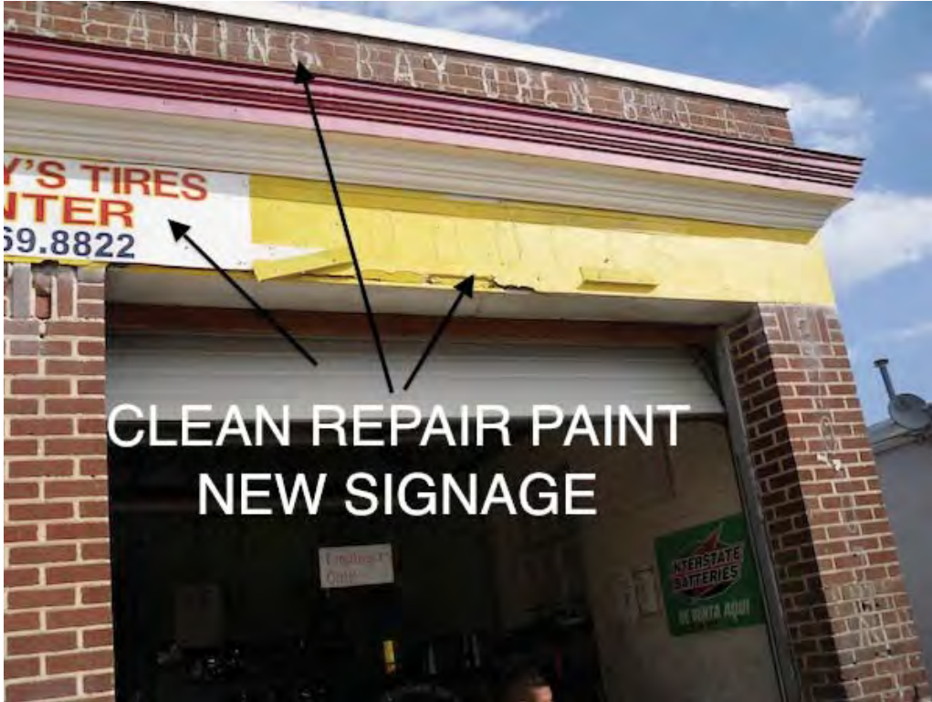
Photo 5. Facing above garage doors.
