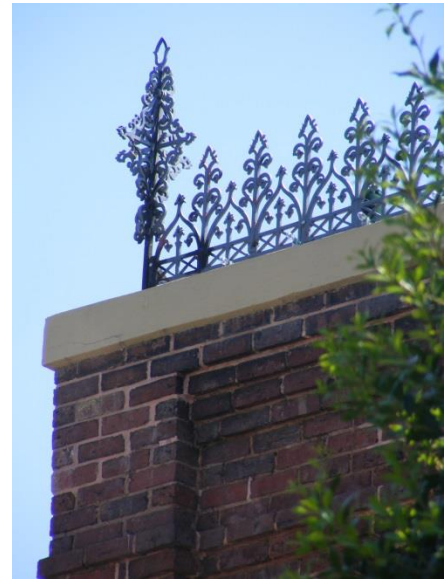
Architectural metal. 15 SE Court Sq
