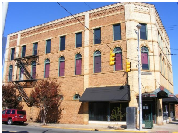
Exterior fire escapes. 200 N Main St
