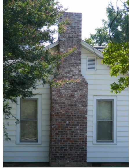
Chimney. 304 W Elm St
