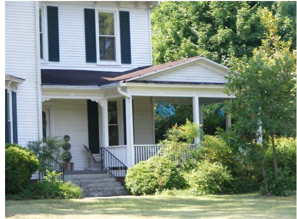
Porch, deck and steps. 312 W Elm St
