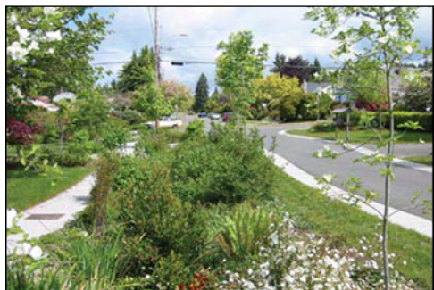
Figure 6(o): Landscaping used on the Sea Street in Seattle, Washington shows how stormwater treatment can be tied to aesthetically pleasing plantings 7 .
