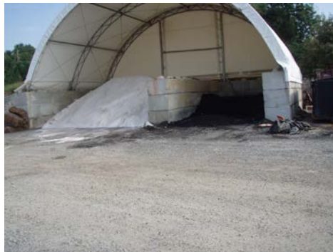
Salt Storage at Public Works
