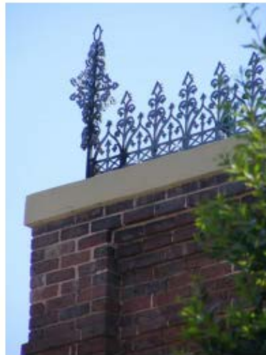
Architectural metal. 15 SE Court Sq
