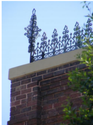
Architectural metal. 15 SE Court Sq
