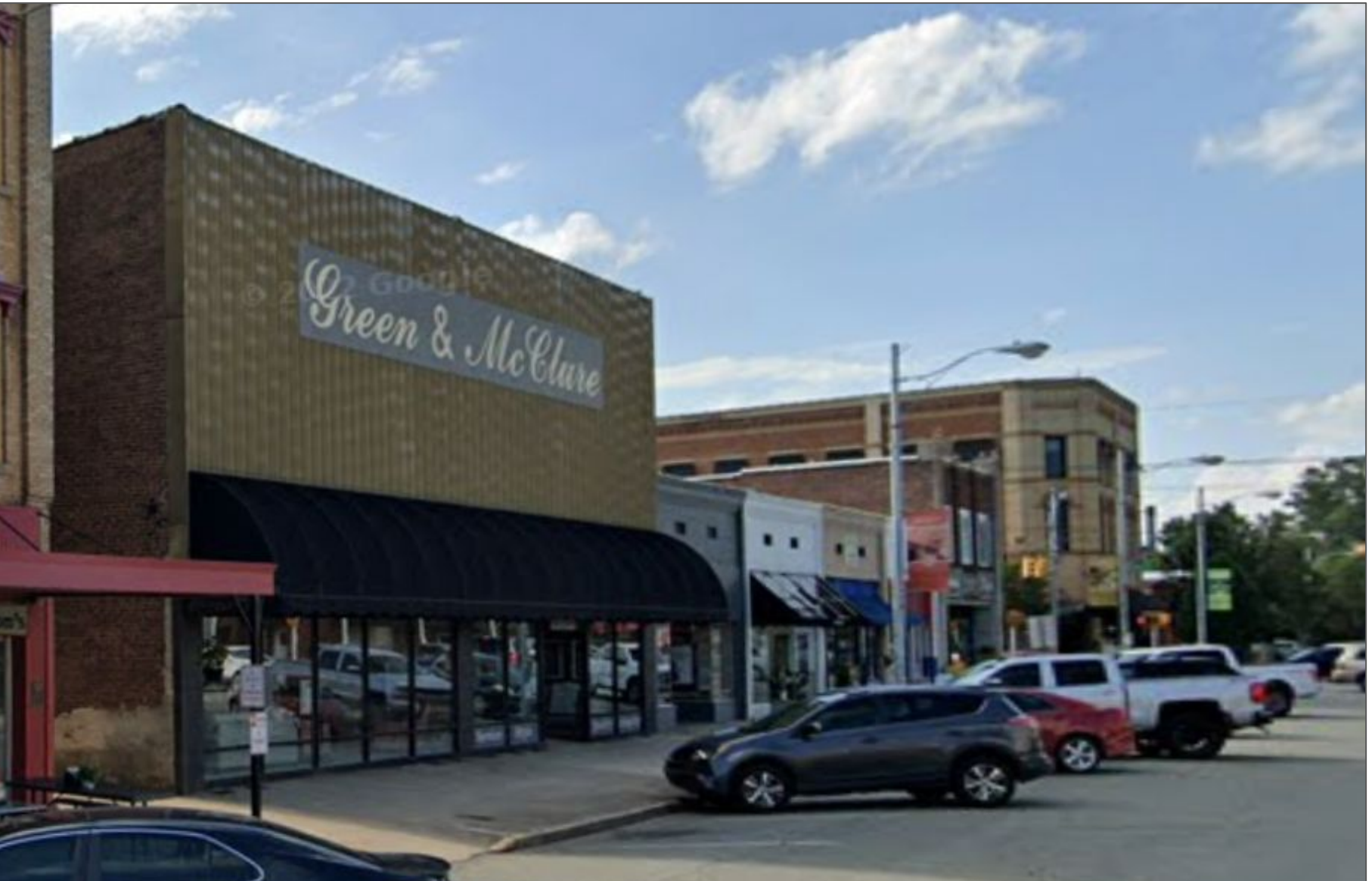
Mid-Century West Facade (prior to panel removal in 2023)
