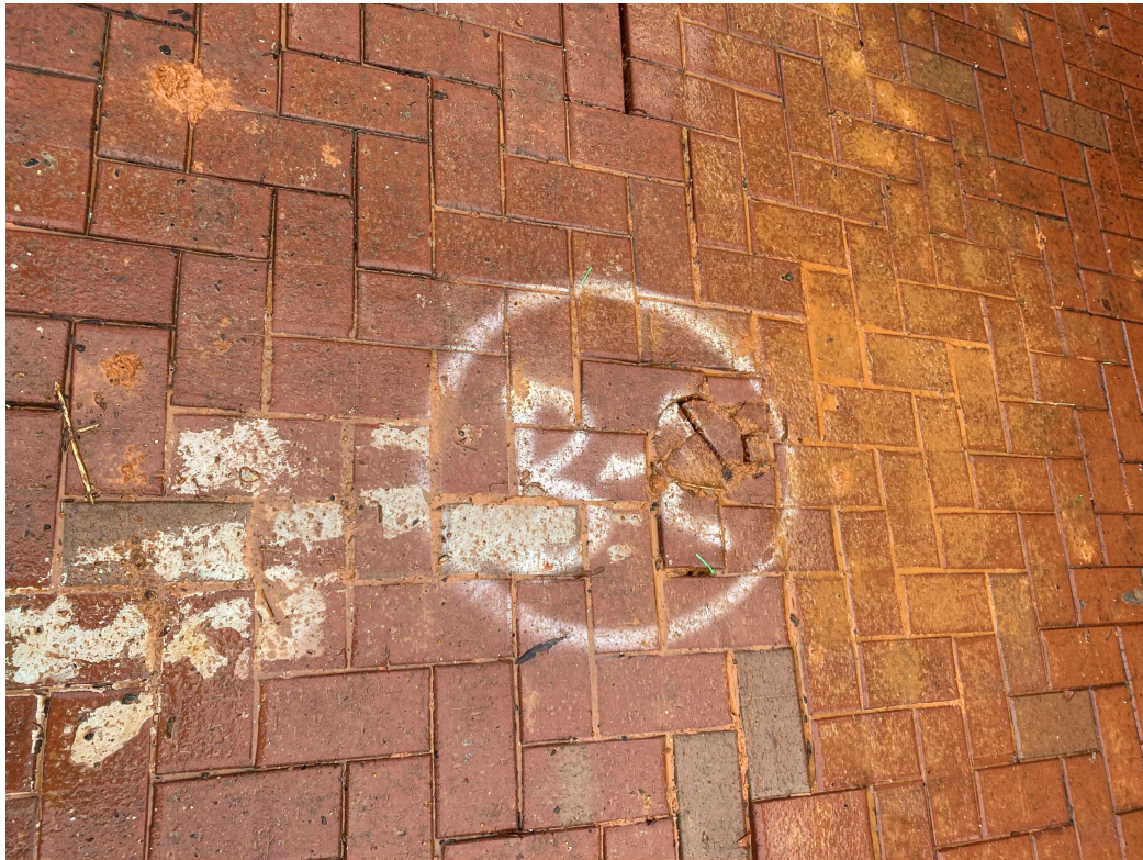
Photo 2 – Boring Abandoned after Sampling
