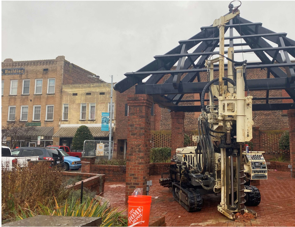
Photo 1 – Drill Rig Set Up at B-1
